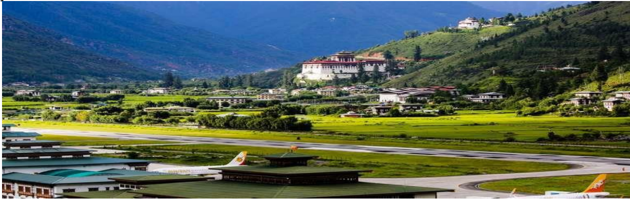
Paro International Airport
